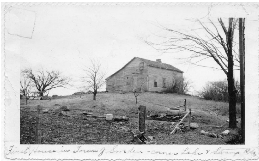
Fig. 9 This view is from the east shoulder of Lake Road (Route 19), looking to the southeast.
