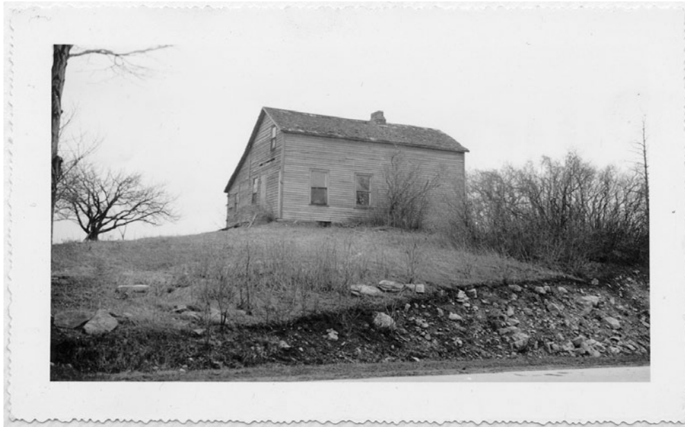
Fig. 8. This view of the same building is from Lake Road (Route 19) looking mostly eastward. The road running left to right at the bottom is Lake Road.
